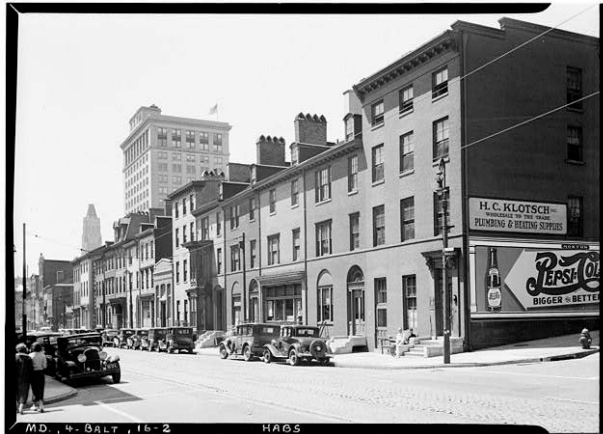
Waterloo Row, 606-628 North Calvert Street 339
