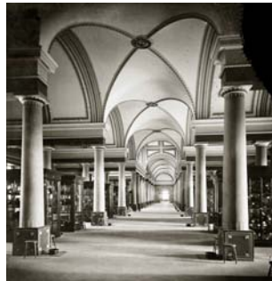
Old Patent Office Model Room with Vaulted Ceiling 362
