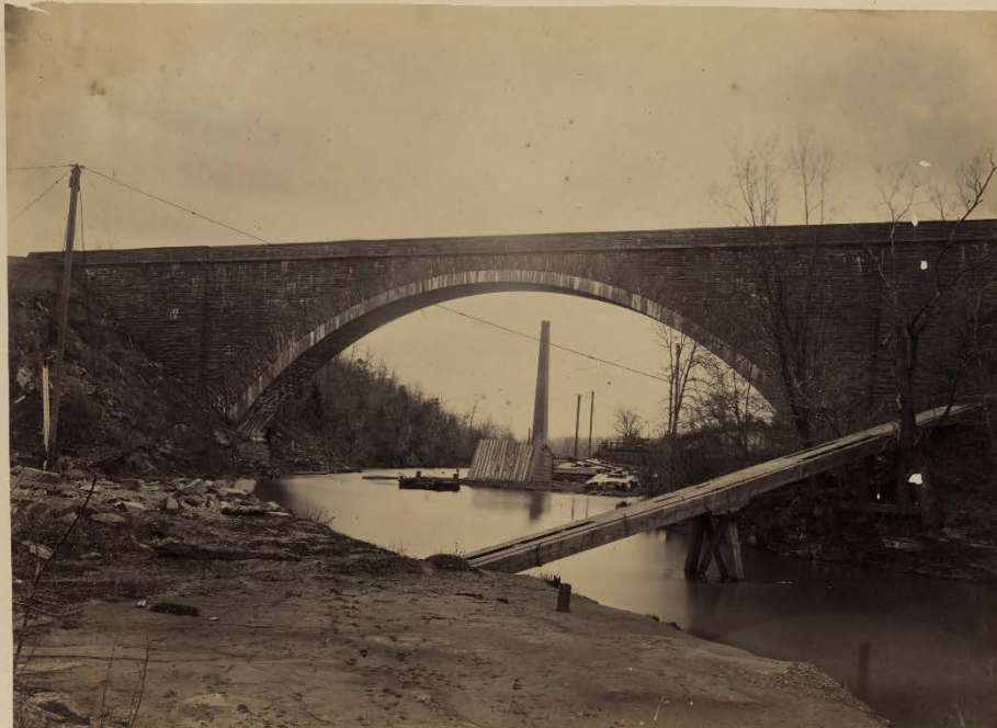
No. 255. - DISTANT VIEW OF UNION ARCH, WASHINGTON AQUEDUCT. Built by Gen. M. C. Meigs. Span of 220 feet.
