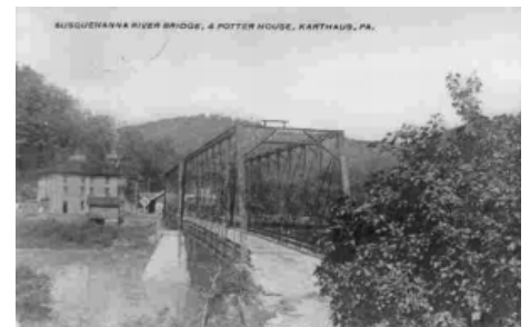
Figure 12: Bridge over Susquehanna River in Karthus, PA
