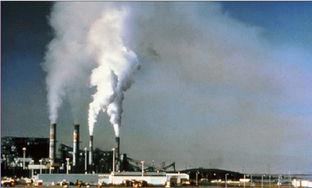
Photo was taken prior to installation of emission controls equipment for removal of sulfur dioxide and particulate matter. Source: U.S. National Park Service
